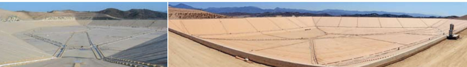
Santa Margarita Water District, Moulton Niguel Water District, South Coast Water District and the cities of San Clemente and San Juan Capistrano partnered to fund the design, construction and maintenance of the Upper Chiquita Reservoir, south Orange County's newest domestic water reservoir. Customers within these service areas will have access to the reservoir's water supply.
