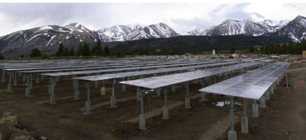
Mammoth Community Water District started construction on a solar power project.
